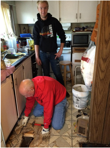
Volunteers Sam Harder and Roger Parsons work to repair a kitchen floor in Lolo this November.
