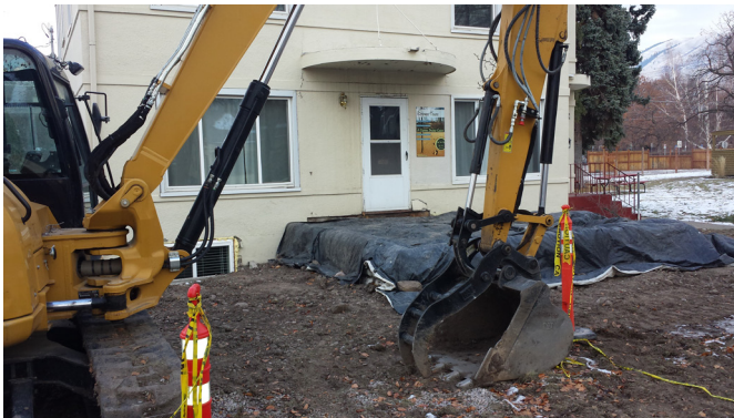
Emmaus house's new porch is under construction and should be completed this spring.
